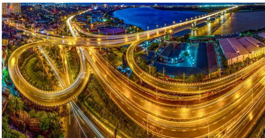
Salon HM - Kim Thanh Dao, Vietnam, Bridge roundabout
